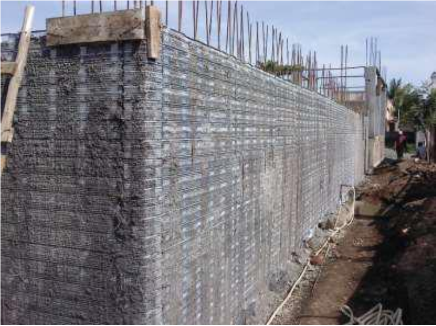
Monolithic Construction With Structural Stay-In-Place CR Steel Specially Designed Formwork System (Coffor)
